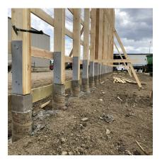
• Grade beams, we also build pole sheds on grade beams for clients that don't want wood in the ground and want the extra strength and security that concrete supplies
